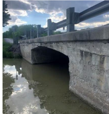
Northeast abutment, looking East
