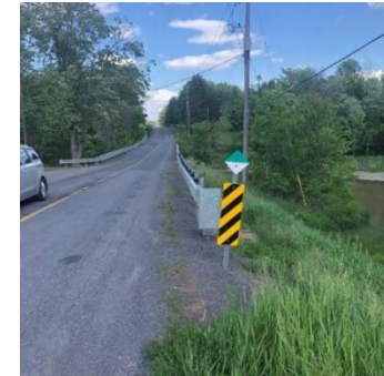
Southwest End of Guard
