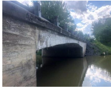
North Side, Underside and West Abutment
