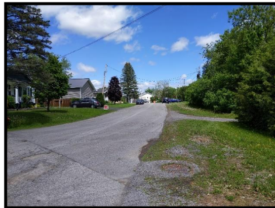
Image 4: Disturbed Lands (May 28, 2022; Facing Northeast)
