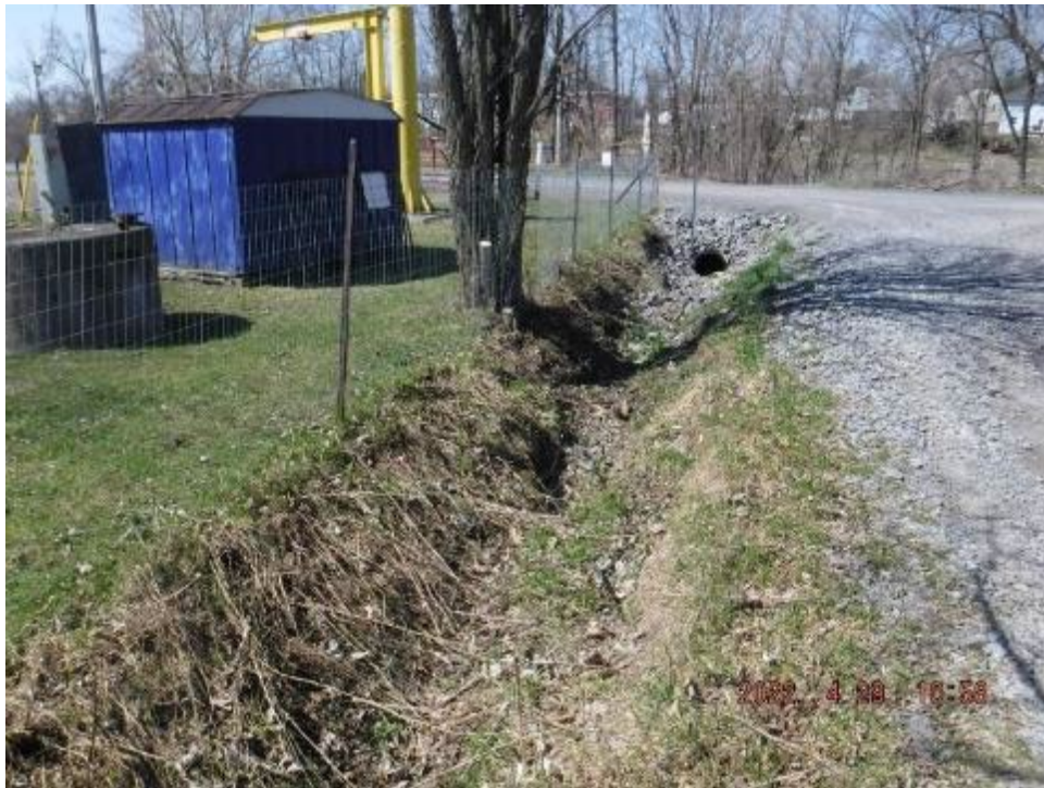
Photo 3: Looking downstream at the south ditch from Concession 5 Road (April 29, 2022)
