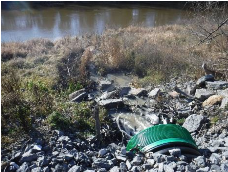
Photo 15: Connection of Unnamed Tributary to South Nation River (November 24, 2021)
