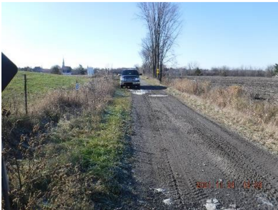
Photo 5: Looking downstream at the absent south ditch in front of the site (November 24, 2021)
