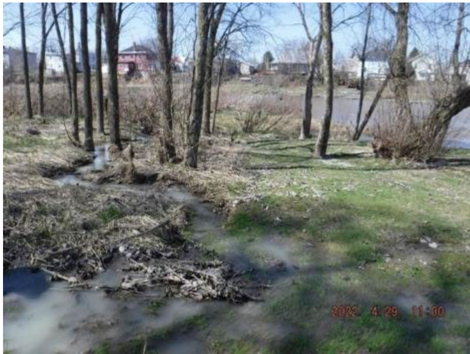
Photo 8: Looking downstream from Pitch Road towards the river and the lack of defined channel of the north ditch (April 29, 2022)
