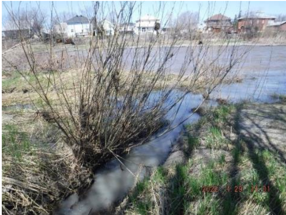
Photo 6: Connection of the north ditch and the river (April 29, 2022)
